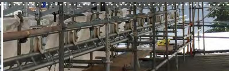
The roof enclosure was moved on rails using muscle power. ⤴
