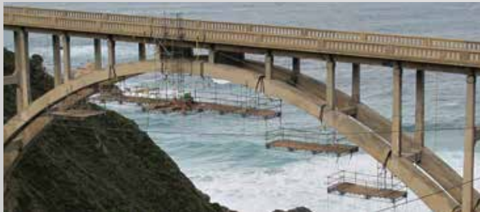
Rocky Creek Bridge, California | Maintaining iconic Pacific Coast landmark | Engineering, QuikDeck ® Suspended Access System
